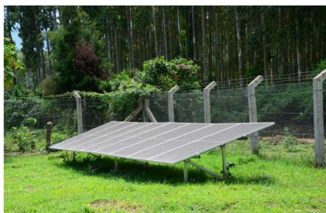
Solar power grid at Kiboota Health Centre III to enable pumping of water for use at the facility
